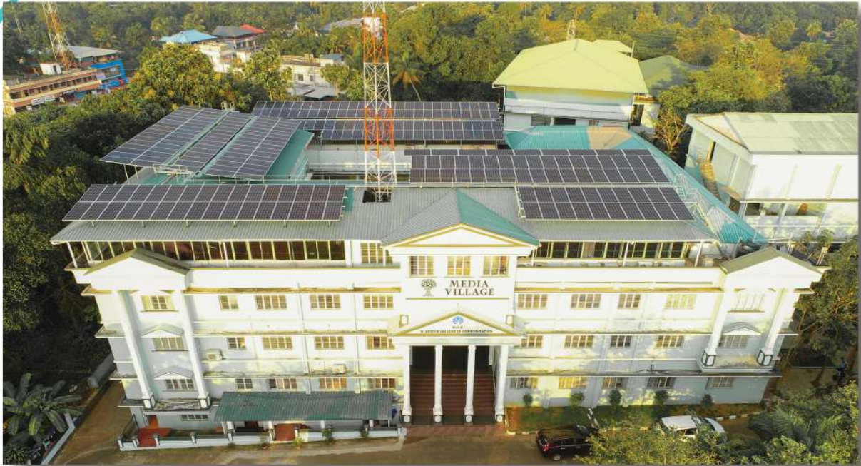
100 kW ON-GRID SOLAR SYSTEM AT MEDIA VILLAGE CHANGANACHERRY
