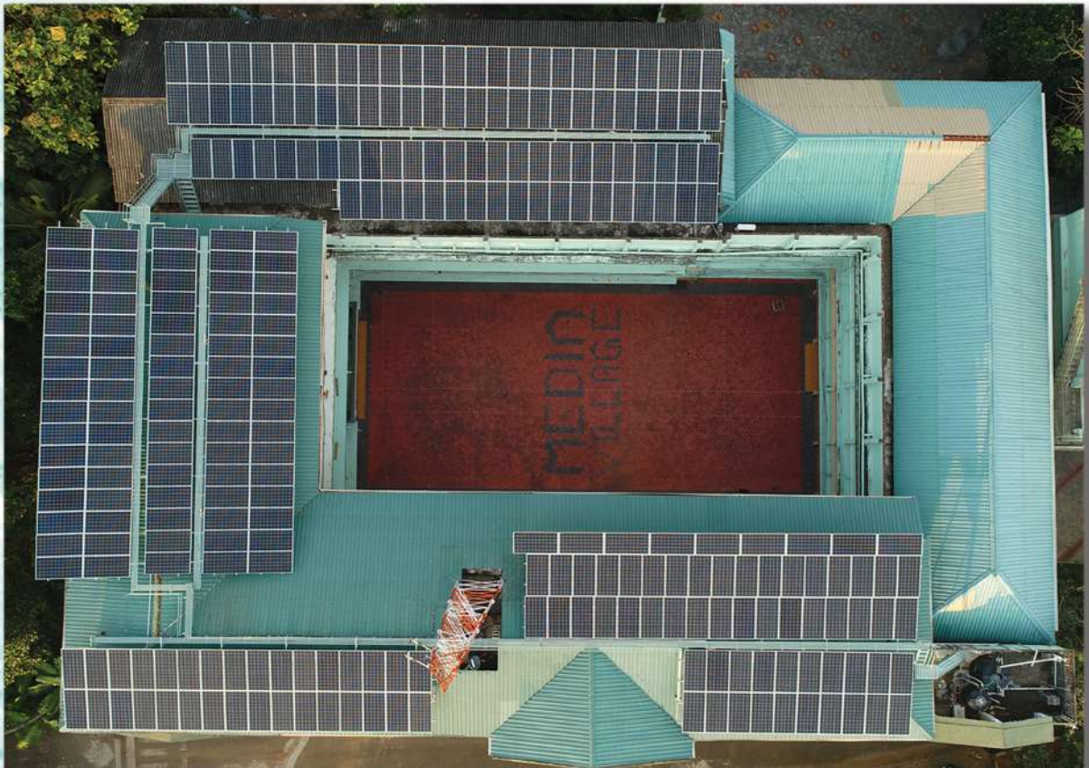
100 kW ON-GRID SOLAR SYSTEM AT MEDIA VILLAGE CHANGANACHERRY
