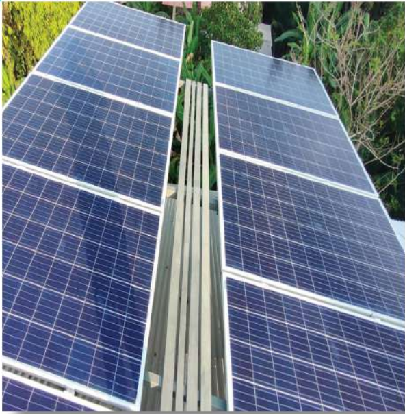
3 kW ON-GRID SOLAR SYSTEM AT CHERUPERIL TRADERS, THIRUVALLA
